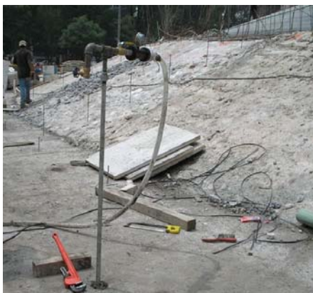
Fig 14, Water injection into the soil, Santoyo et al (2005)
