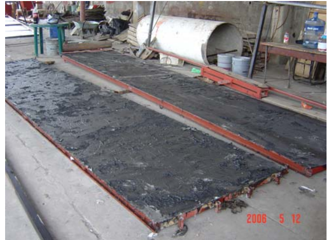
(a) Preparation of panels
