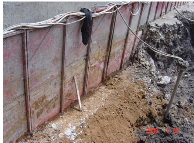
(b) Panels after installation
