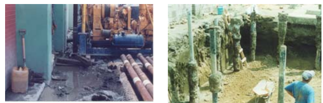
Fig 7, Micropiles under construction in Mexico City
